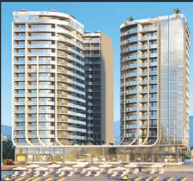
ELT BUILDING - MARINA CLUB
